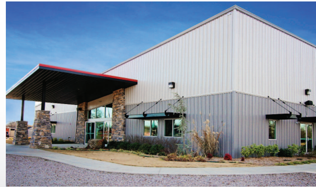
The BOD-TV Church Roland, Oklahoma B & B Welding, Inc., Builder
